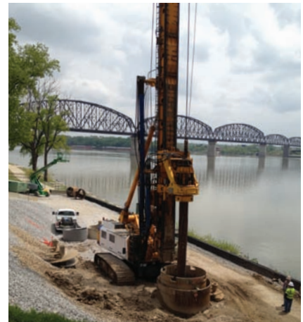
The drilling of 50-foot deep test shafts on the Indiana shore across from Louisville is one of the first large pre-construction operations for the $2.3 billion Ohio River Bridges Project. A new six-lane Downtown Crossing bridge between downtown Louisville and Jeffersonville along with another new bridge six miles upstream at Prospect, Ky., are to be open for traffic in 2016. An official ceremonial start of construction is planned for July 1.
