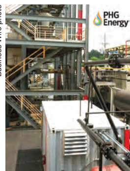
PHG Energy integrated GE's heat-to-power technology (white unit in foreground) into an existing gasification system installed to provide producer gas for a brick kiln operation in Gleason, Tenn.
