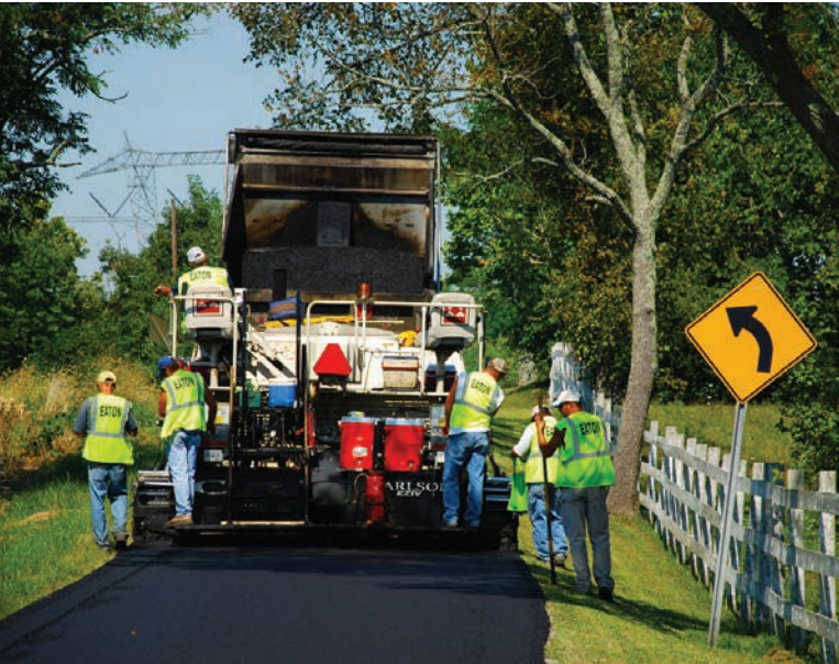
A road construction crew paves a scenic Kentucky roadway with asphalt. The Kentucky Transportation Cabinet invests in hundreds of paving projects each year.
