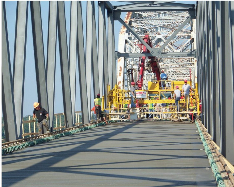
These shots, from May 2012, show the concrete deck being poured on a new, replacement span of the Eggners Ferry Bridge on Kentucky Lake. The original span was knocked out by a cargo vessel in January 2012.
