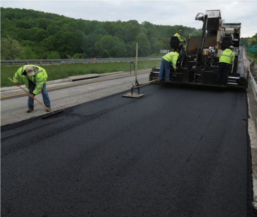
Crews apply asphalt resurfacing along Interstate 64 this past summer in Bath and Rowan counties. The project was funded by the Kentucky Transportation Cabinet's annual maintenance budget for major routes.
