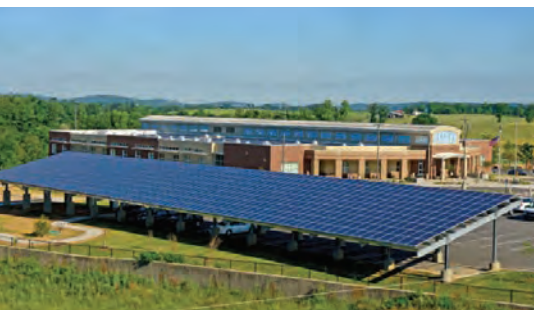
Richardsville Elementary in Bowling Green was the first net-zero school in the nation. It generates at least as much electricity and other power as it uses.
