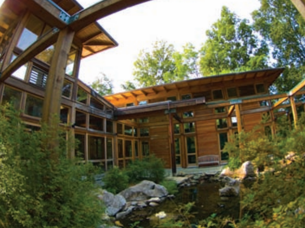
The Visitor's Center at Bernheim Arboretum and Research Forest in Nelson and Bullitt counties received the platinum award from the U.S. Green Building Council LEED for its design featuring passive and active solar design, geothermal exchange, and the use of recycled building materials.
