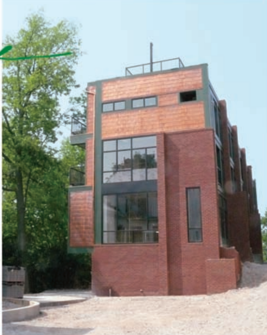
First phase while under construction and before any landscape or driveway improvements. Building exterior features brick veneer with copper shingles and downspouts.
