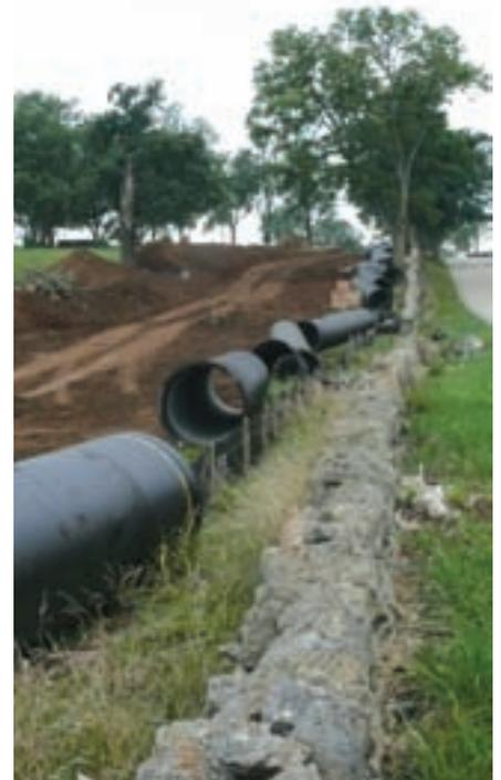
Above: Pieces of 42-inch pipe lay along a roadway for construction of a Kentucky American Water Co. water line from the Kentucky River in Owen County to Lexington.
