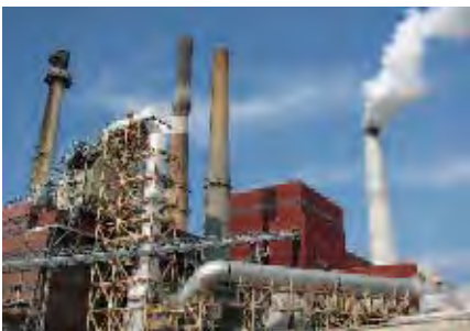
The E.W. Brown Generating Station on Herrington Lake in Mercer County includes three coal units totaling 700 megawatts, supplemented by six natural gas/fuel oil turbine units that can generate 768 megawatts, and the 24 megawatt Dix Dam Hydro Plant built in the 1920s.
