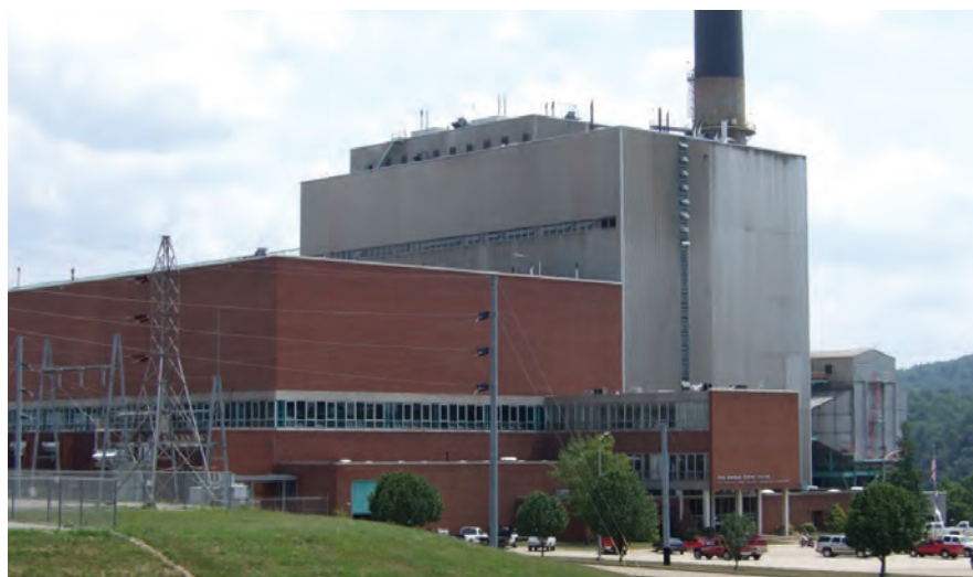
East Kentucky Power Cooperative's coal-fired 225-megawatt Cooper Station Unit 2 in Somerset, which went online in 1969, underwent a flue gas desulfurization, selective catalytic reduction and pulse-jet fabric filter retrofit to meet modern air emission standards.
