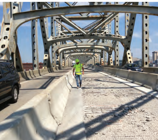
Work in summer 2017 to replace the deck of the Brent Spence Bridge as well as improve lighting and drainage brought lane closures that worsened delays already estimated to total 3.6 million hours annually.
