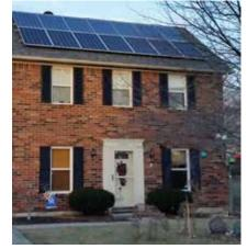
A small individual solar power system such as this one typically produces between 3,000 and 3,500 watts of power. Panels have a life expectancy, according to homeadvisor.com, of 14-17 years for thin-film, 23-27 years for polycrystalline and 25-35 years for monocrystalline.
