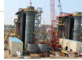
A 640-megawatt natural gas-fired Cane Run Generating Station unit, shown during construction in western Louisville, went online in 2015. Replacing coal-burning units built in the 1950s, it generates electricity with gas turbines, and then recycles exhaust heat to generate steam and produce additional power.
