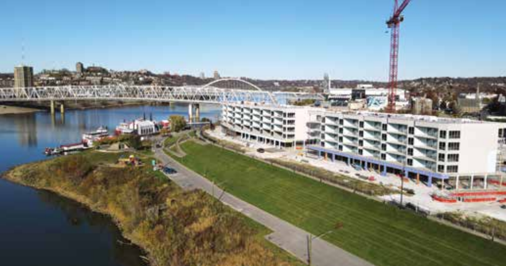
Ovation project apartments nearing completion at the confluence of the Licking and Ohio rivers in Newport face the Cincinnati skyline directly across the river.
